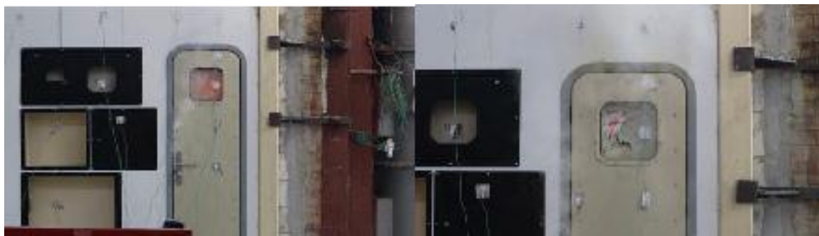
Fig. 3a, b. Door window under fire action.
