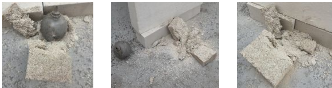
Fig. 4. Degradation of brittle matter as a boundary phenomenon - hemp with cement.
